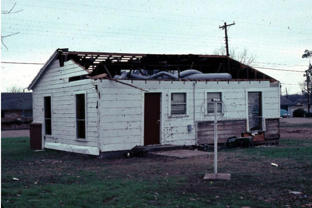
**Figure 4. The roof on this house was not anchored very well and was uplifted during peripheral winds in the Mesquite, TX tornado on December 13, 1994. wind velocities of less than 100mph (161 km/h) can cause such residential damage.**
