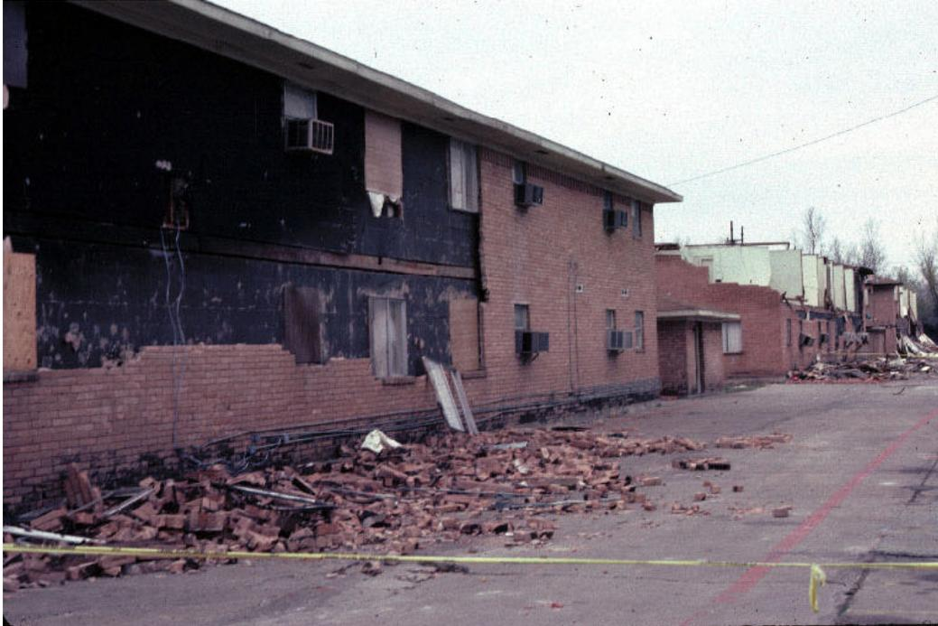
**Figure 6. Damage to a two-story brick veneer wall in the Mesquite, TX tornado. There were no brick ties to anchor the wall to the wooden frame. The wall toppled on the leeward or "suction" side.**
