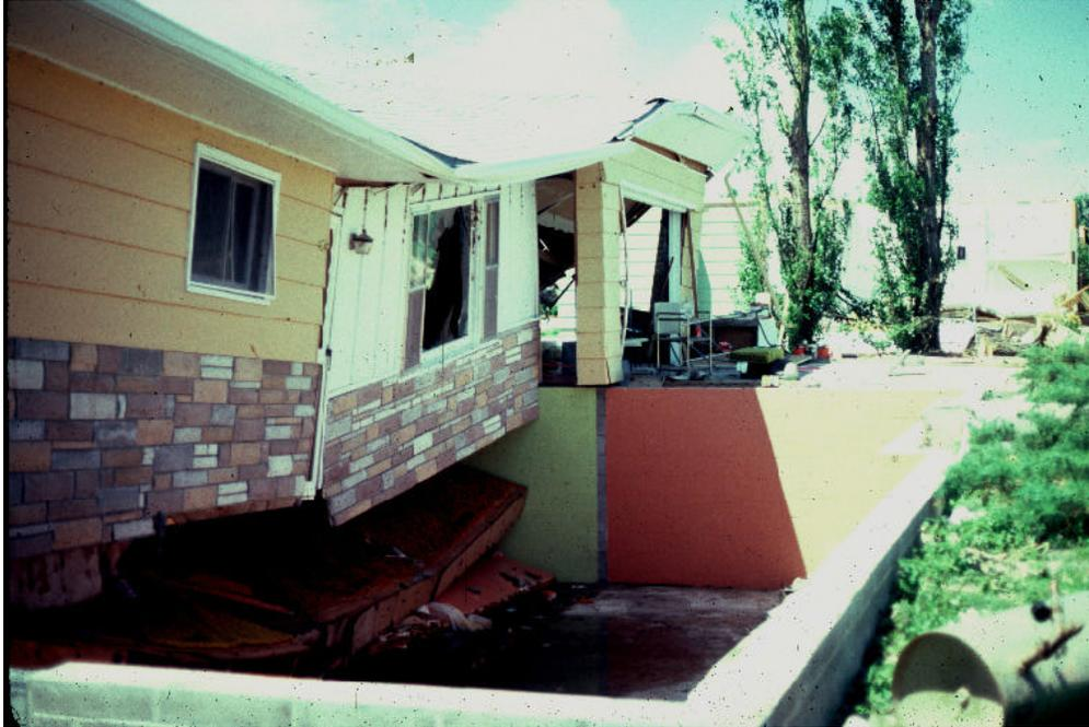
**Figure 3. Lateral displacement of this unanchored home during the Grand Island, NE tornado caused the wooden floor structure to lose support and fall into the basement. Lack of damage to the surrounding trees and roof shingles indicated house movement occurred at wind velocities of probably less than 100 mph (161 km/h).**
